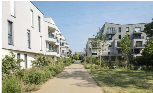
Figure 7 écoquartier Centre Sainte-Geneviève
